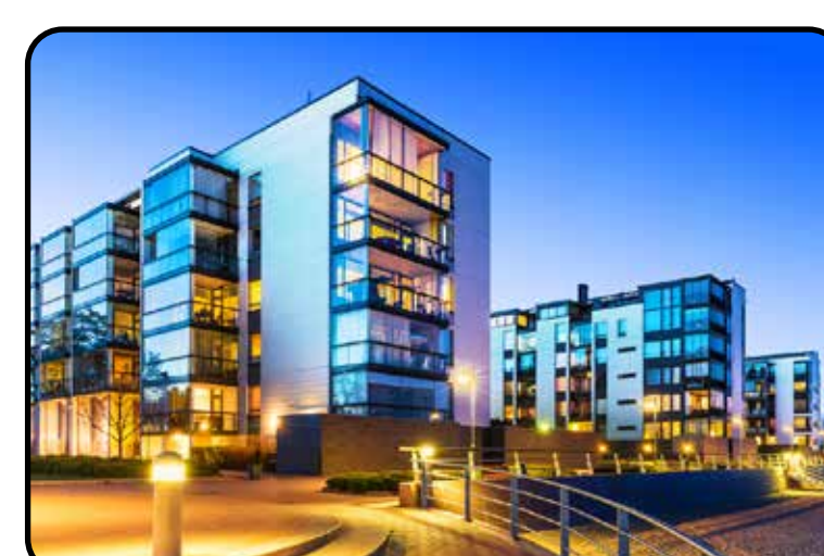
Building Security Control
